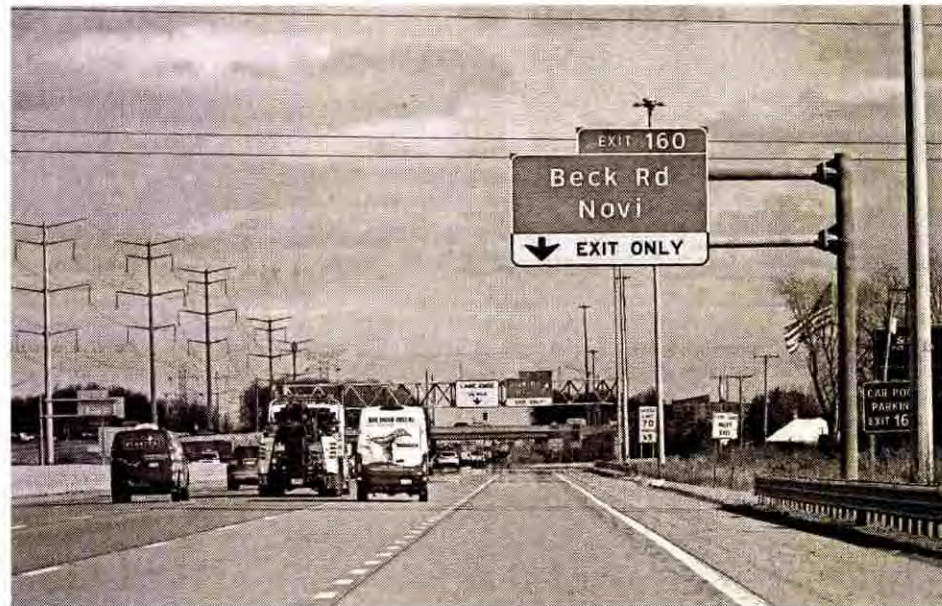
I-96 eastbound near Beck Road. Roadwork will begin this summer to rehabilitate I-96's breakdown lanes and to eventually add a rush-hour lane near its median.
