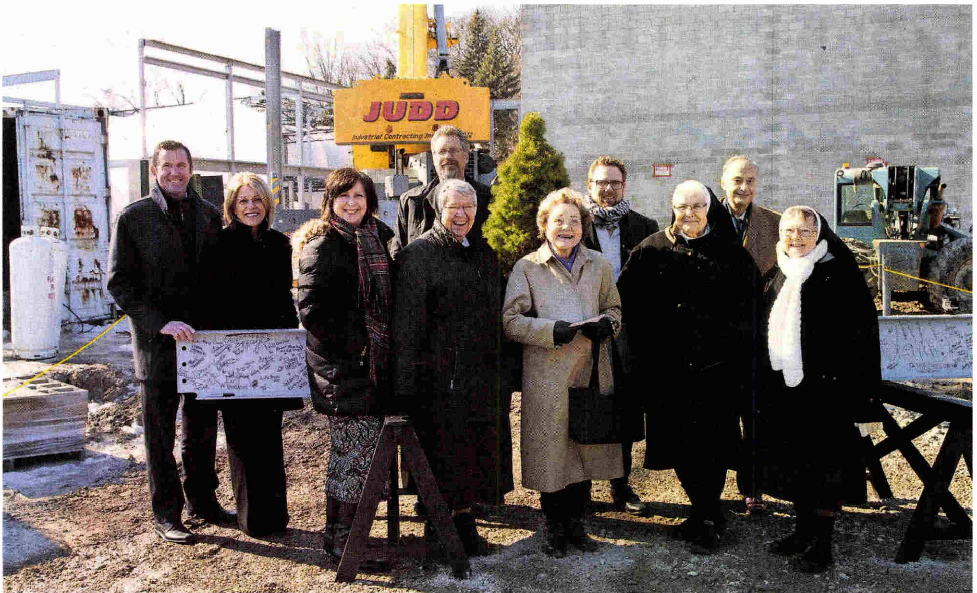
Madonna University supporters and Felician Sisters attend the ceremony of raising the final beam for the university's welcome center. COURTESY OF MADONNA UNIVERSITY
