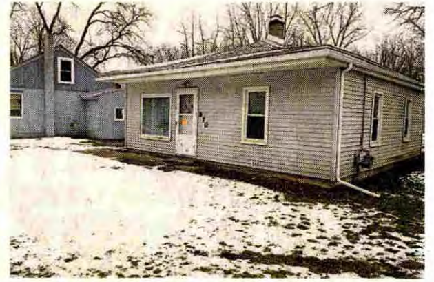
The owner of this home at 870 Lotz Road in Canton has been given an extension of time to fix the mold problem in the home or raze it. HOMETOWNLIFE.COM FILE
