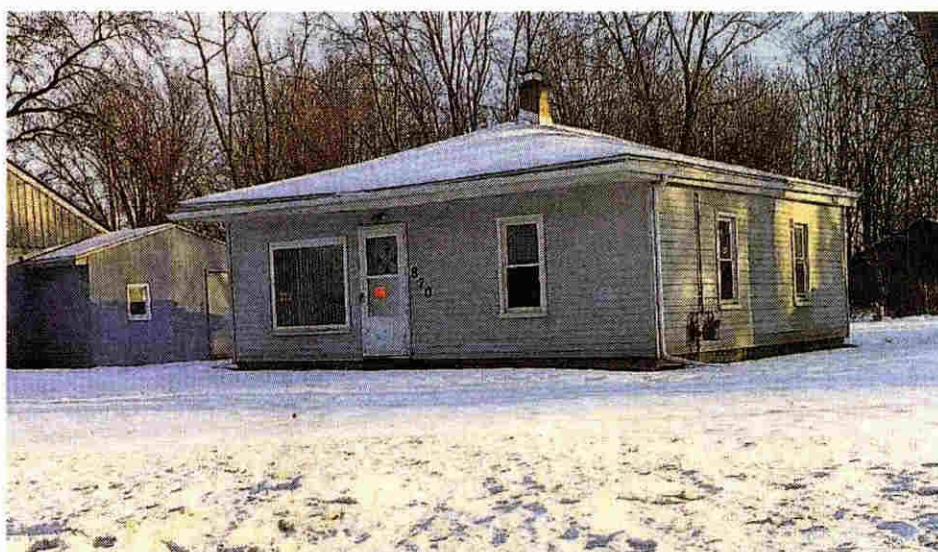
The vacant home at 870 Lotz Road in Canton has a date with the wrecking ball, but its owner is fighting the township over the issue. ED WRIGHT/HOMETOWNLIFE.COM
