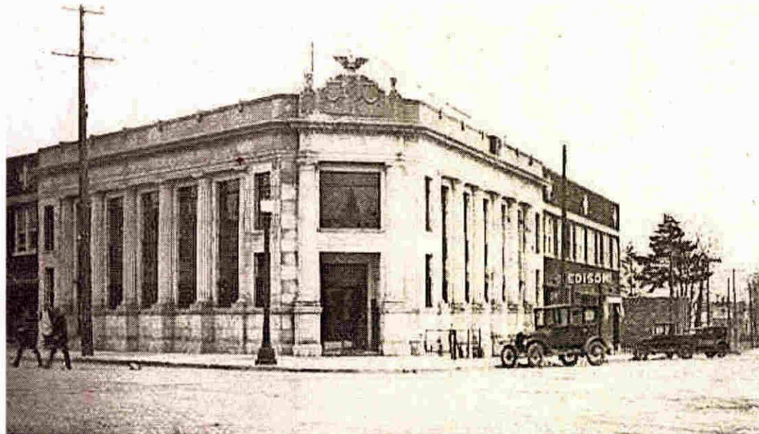
Farmington State Savings Bank (now the Village Mall) opened at Grand River and Farmington Road on March 18, 1922. The lobby was marble and walnut and the vault door weighed more than 10,000 pounds. GLP Financial Group recently purchased the building from Farmington Holding Company, which has managed the property since 1975 after the Warner family purchased it back in the 1970s.
