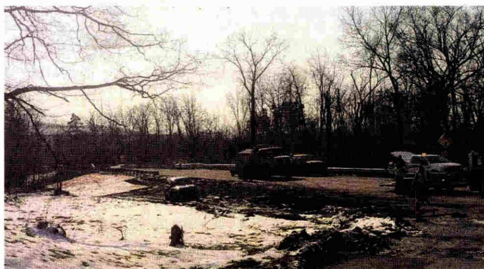
Members of the Wayne County Roads Commission remove barrels and barriers from the now-open Lilley Road bridge. ED WRIGHT/HOMETOWNLIFE.COM
