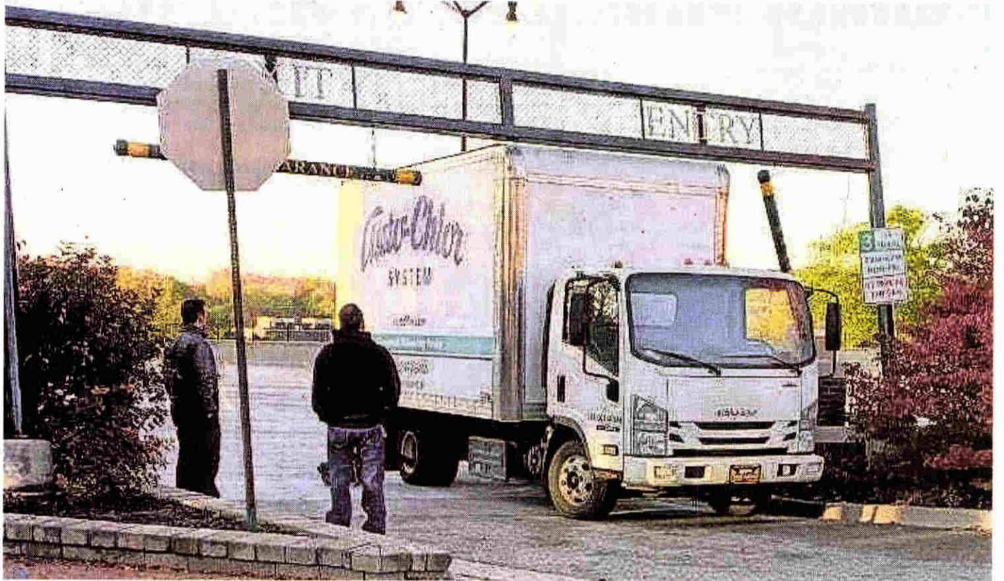
Less than 24 hours after the parking deck renovation was completed, a truck that was too tall jolted the signs above the entry ramp. No one was injured in the incident, and the parking deck reopened after a few hours. COURTESY OF NORTHVILLE DDA
