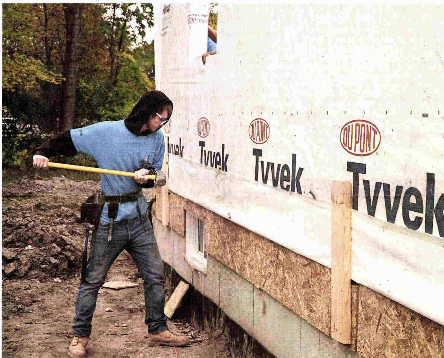
High school student Kirk Mason uses a sledgehammer to level a home's wall after it has been lifted into place during the construction technology class at Wayne-Westland Community Schools. PHOTOS BY JOHN HEIDER/HOMETOWNLIFE.COM
