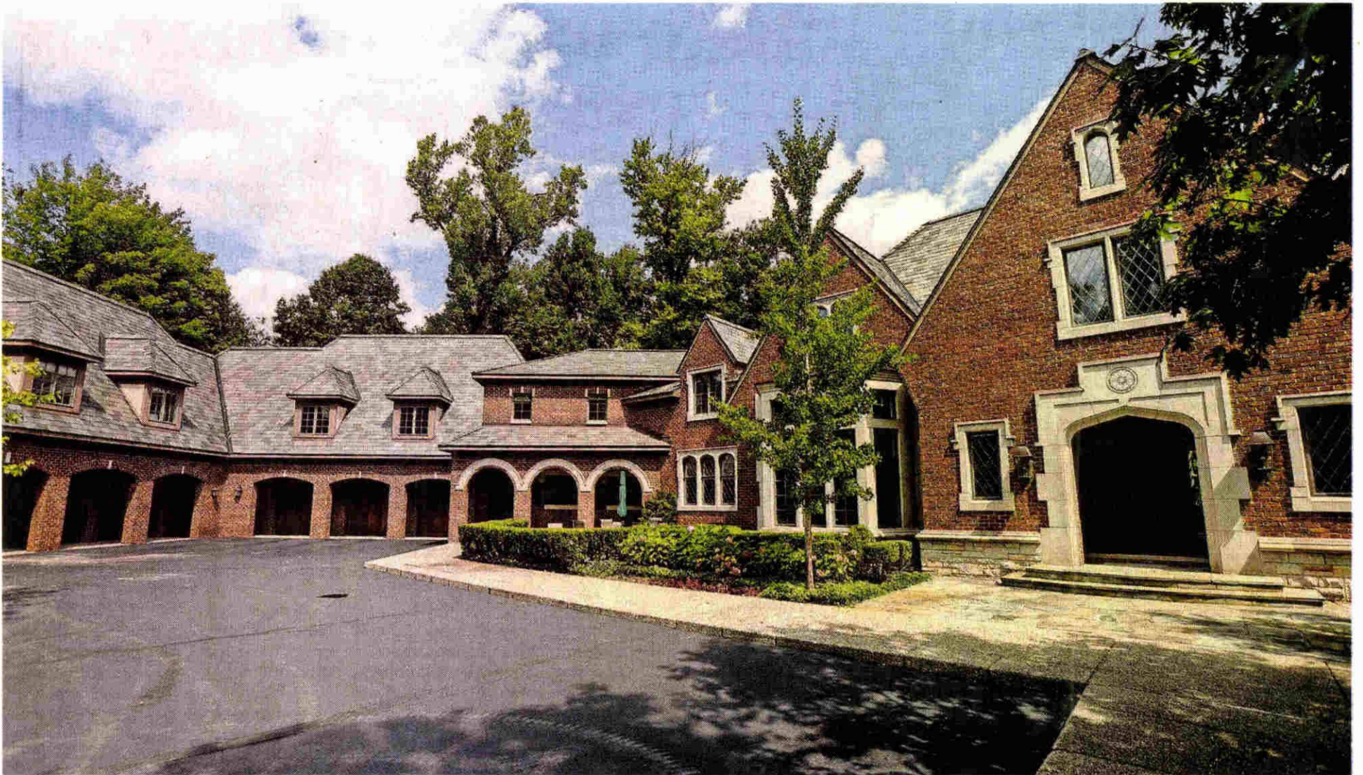
This English manor-style home is brick with limestone trim and features a six-car garage. The roof is slate, with peaks, valleys and dormers. ERIC SEALS/DETROIT FREE PRESS
