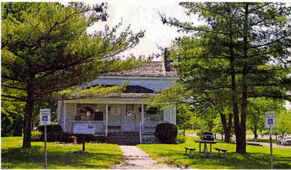
The historic Cranson-Hinbern House will likely see a new roof this summer. PHOTOS BY SHELBY TANKERSLEY/HOMETOWNLIFE.COM
