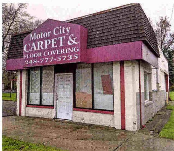
A brewery is proposed for this location on Seven Mile between Inkster and Harrison in Livonia.
