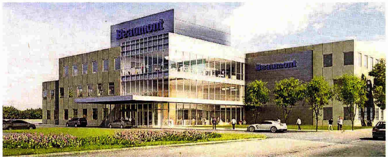
Beaumont Health will open a new medical facility in 2020 near Seven Mile and Interstate 275 in Livonia.
