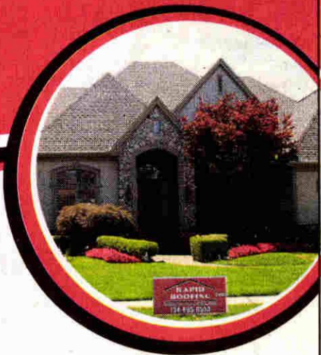
Actual Rapid Roofing Completed Project
