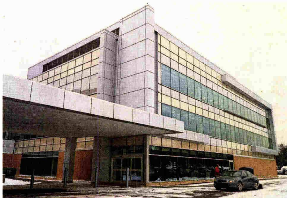
The hospital will open the $160 million expansion throughout the month. City council approved the project in 2015, and ground was broken in 2016.
