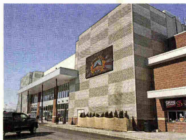
Part of the Suburban Collection Showplace's massive expansion connects to the rest of the convention hall at its west end. JOHN HEIDER/HOMETOWNLIFE.COM
