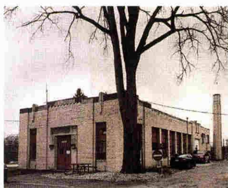
Newburgh Mill, located on Hines Drive at Newburgh Road. BILL BRESLER | HOMETOWNLIFE.COM
