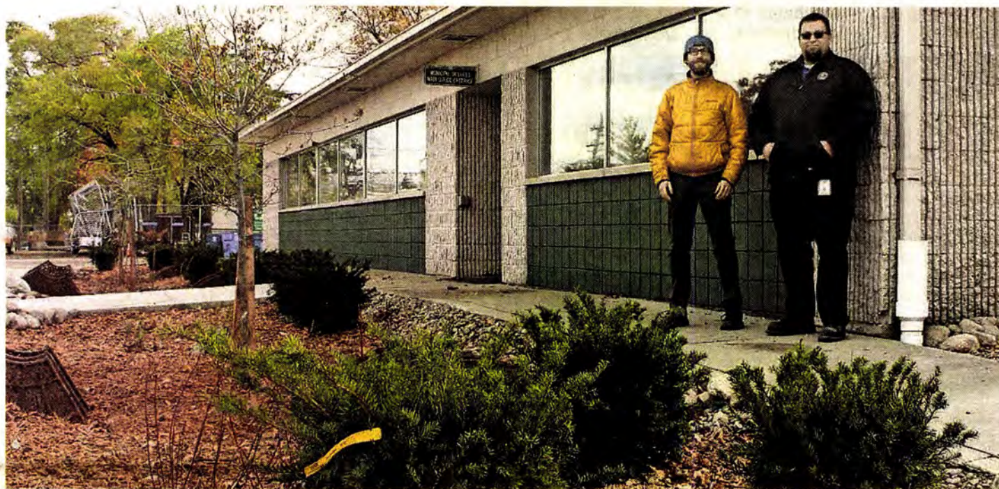
Matthew Bertrand and Adam Gerlach teamed to kick-start a flood-eliminating project in front of the Plymouth municipal services headquarters. ED WRIGHT | HOMETOWNLIFE.COM
