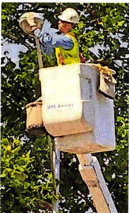
A DTE worker converting a mercury vapor street light to LED. FILE PHOTO
