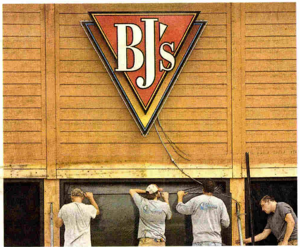
Construction workers install glass at BJ's Restaurant & Brewhouse. BILL BRESLER | HOMETOWNLIFE.COM
