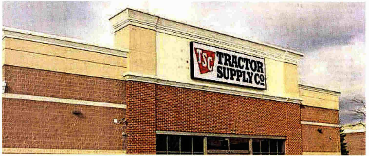
Tractor Supply Co. is expected to break ground on its Canton store as early as August. PHILLIP BOCK | USA TODAY NETWORK — WISCONSIN
