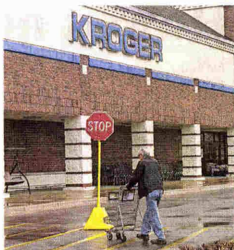
The Kroger store on Haggerty Road in Northville Township has received a $3.5 million makeover. BILL BRESLER | HOMETOWNLIFE.COM
