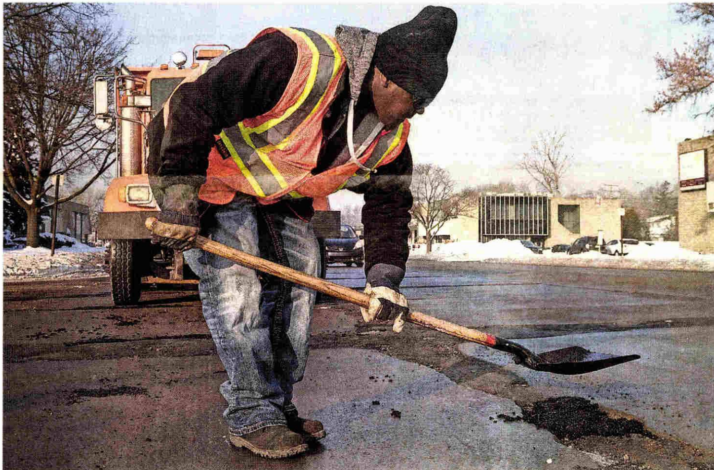
After filling the hole, Daimon Parker tamps down the patch with the back of the shovel blade. He knows the patch is temporary. Michigan's freeze-thaw cycle means that road crews never run out of work. BILL BRESLER | HOMETOWNLIFE.COM
