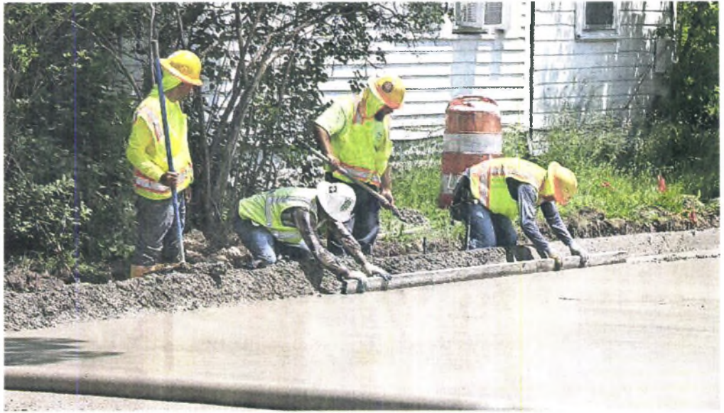
Westland Department of Public Services workers are tackling local road projects.
