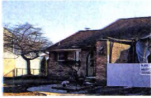
DAVID VESELENAK A fire that started in a garage at this home in the 38000 block of Meeting House Lane in Livonia has been deemed accidental.
