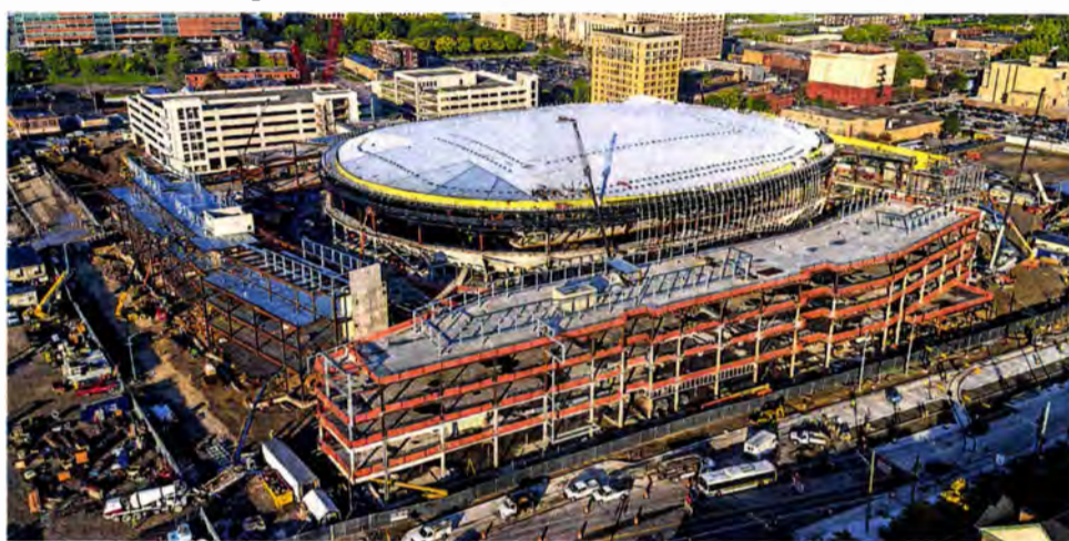
Little Caesars Arena construction, pictured in October 2016 in Detroit.
