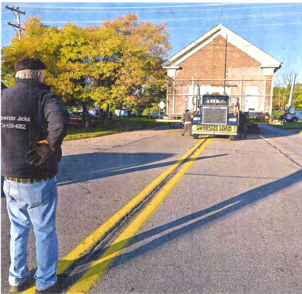
Waiting for DTE to raise the power lines.
