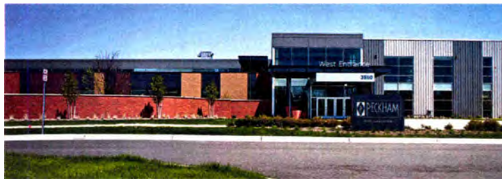
The manufacturing facility of Peckham Industries, Inc. is near the Capital Region International Airport.
