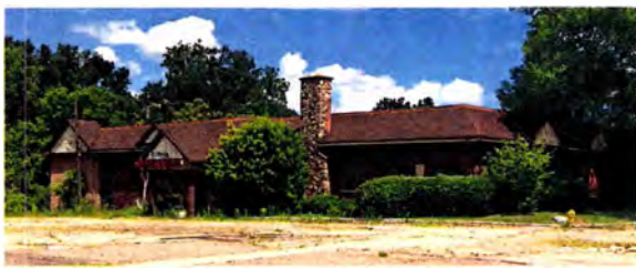
The City of Westland owns the building and Merriman Road frontage of the defunct New Hawthorne Valley.
