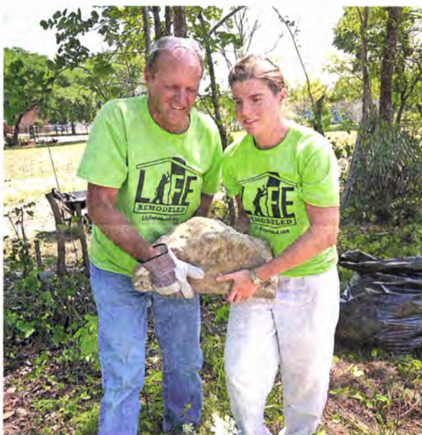
Randy Gasser and daughter Angela Gasser haul a piece of concrete to the curb. They are from Livonia.
