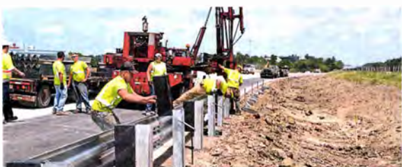
Crews work on replacing a guardrail along I-275.
