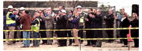
JOHN STORMZAND | STAFF PHOTOGRAPHER Placing of the final beam on the Masco Corporation building construction at Schoolcraft College drew applause.
