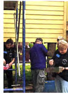
Volunteers mix joint compound for mudding the drywall.
