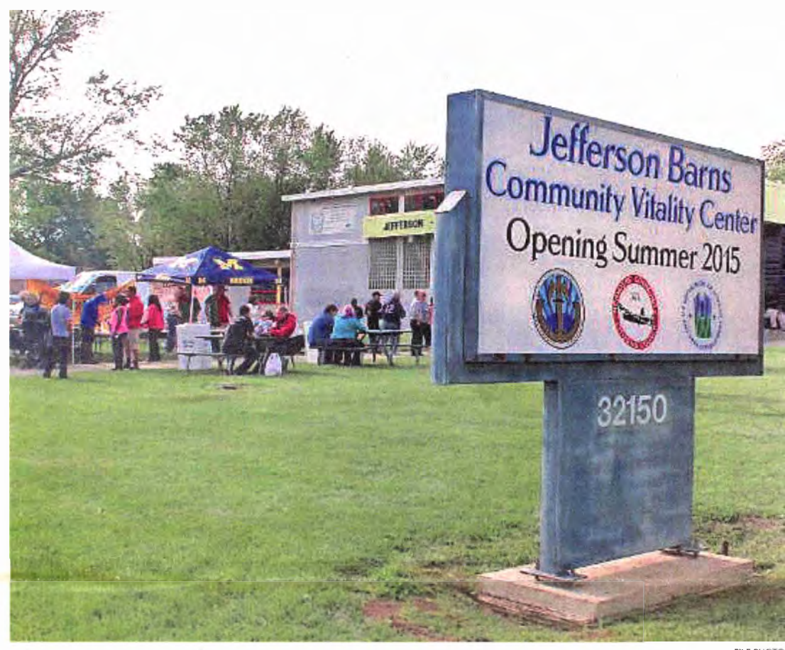
Westland opened the newly renovated Jefferson Barns Community Vitality Center in July 2015 in a vacant elementary school. FILE PHOTO
