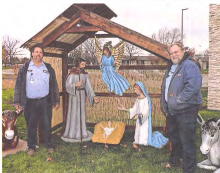
Westland Department of Public Services workers Tom Sharp (left) and Ian Smith are being honored for their efforts building a new manger for the city's Christmas display.
