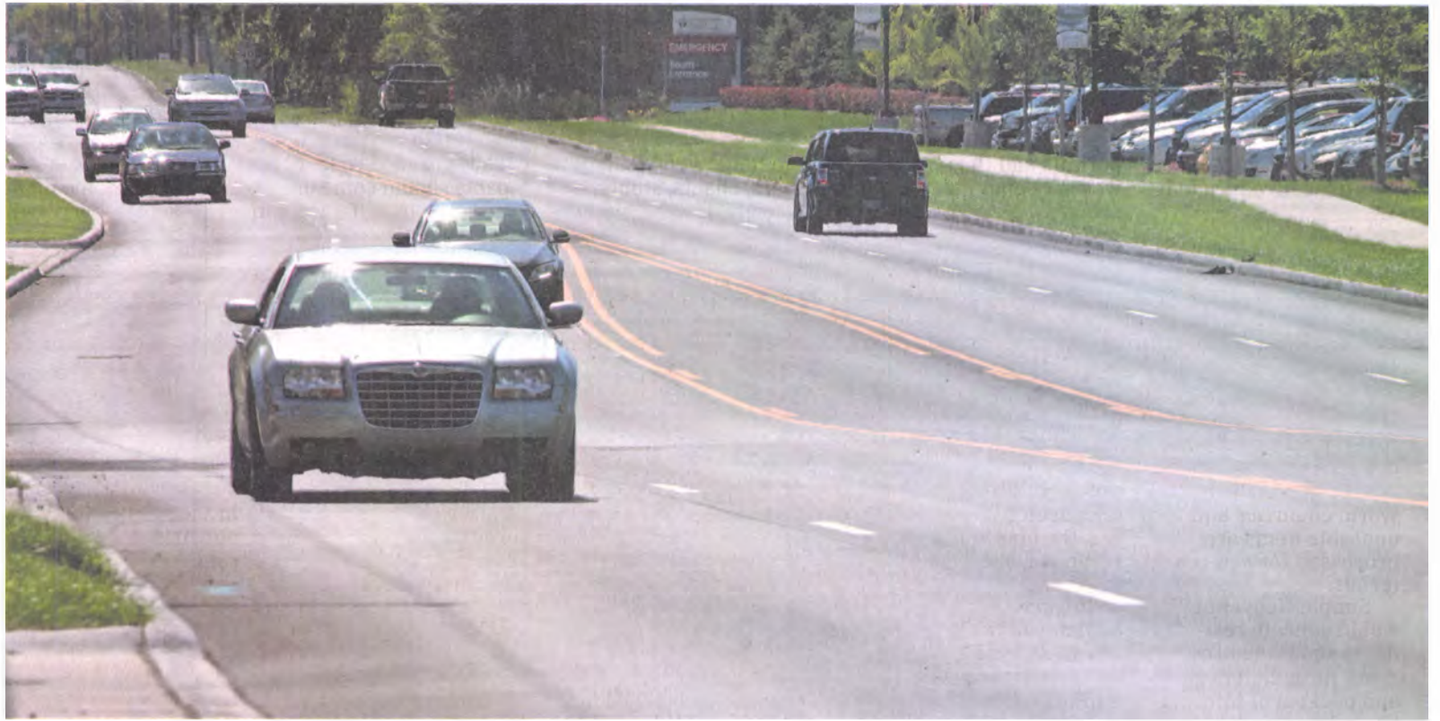
Cars drive on Levan Road on Thursday. The one-mile stretch from Schoolcraft to Five Mile was recently resurfaced.
