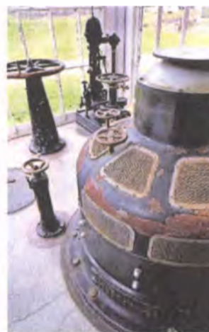
Edison's generator is turned by the water turbine below. Hand wheels raise and lower the gate that controls flow.
