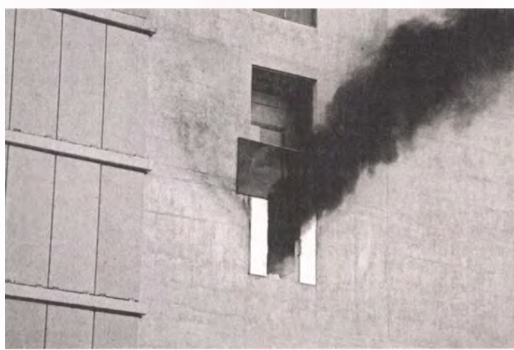
Fire drills are important for all buildings including high-rise structures. GETTY IMAGES
