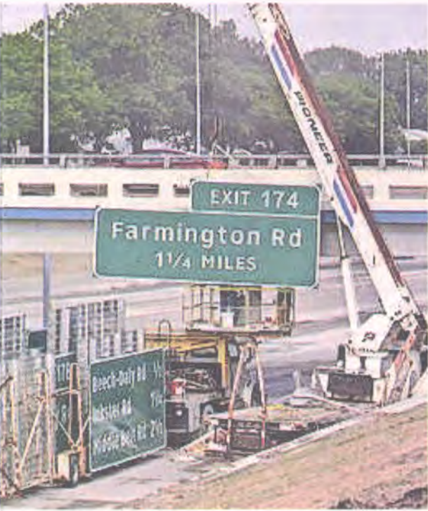
It's been one year since I-96 shut down for reconstruction. Some minimal work will continue this spring on the project, but it will have little impact on drivers.
