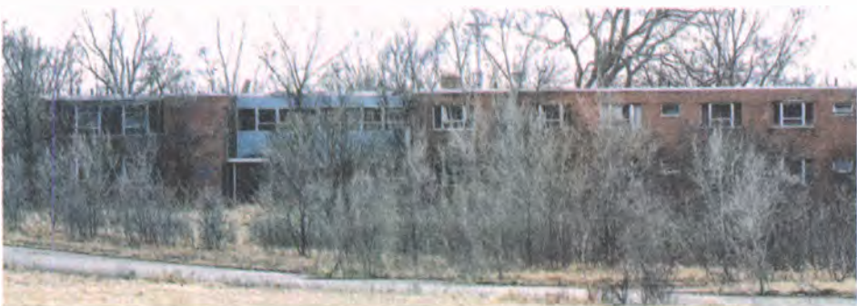
This building, No. 72, at the former Northville Regional Psychiatric Hospital on Seven Mile, is to be torn down soon.
