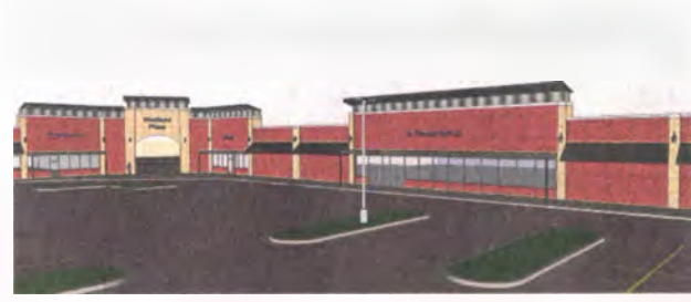
A building to replace the former Marvaso's Italian Grille/Electric Stick is under construction. The entire Westland Plaza will be getting new facades, along with a memorial to fallen Wayne-Westland Firefighter Brian Woehlke.
