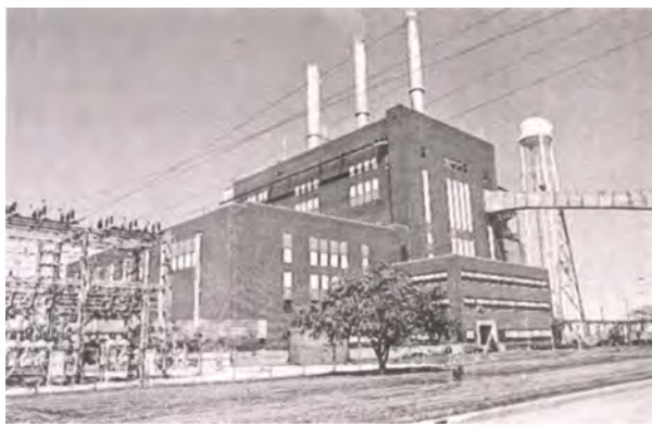
Consumer's Energy J.R. Whiting Generating Complex on an 875-acre site along the Lake Erie shoreline in Erie is one of the smallest coal-fired plants in the company's fleet. It began producing electricity in 1952.
