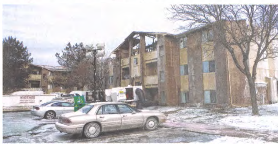
Fire officials and workers were already assessing the damage at Woodland Villa a day after a fire destroyed eight units.
