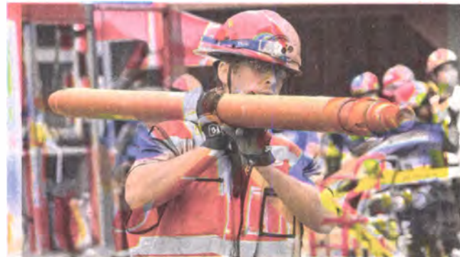
A member of the Urban Search And Rescue team carries adjustable metal struts that will help stabilize the home.
