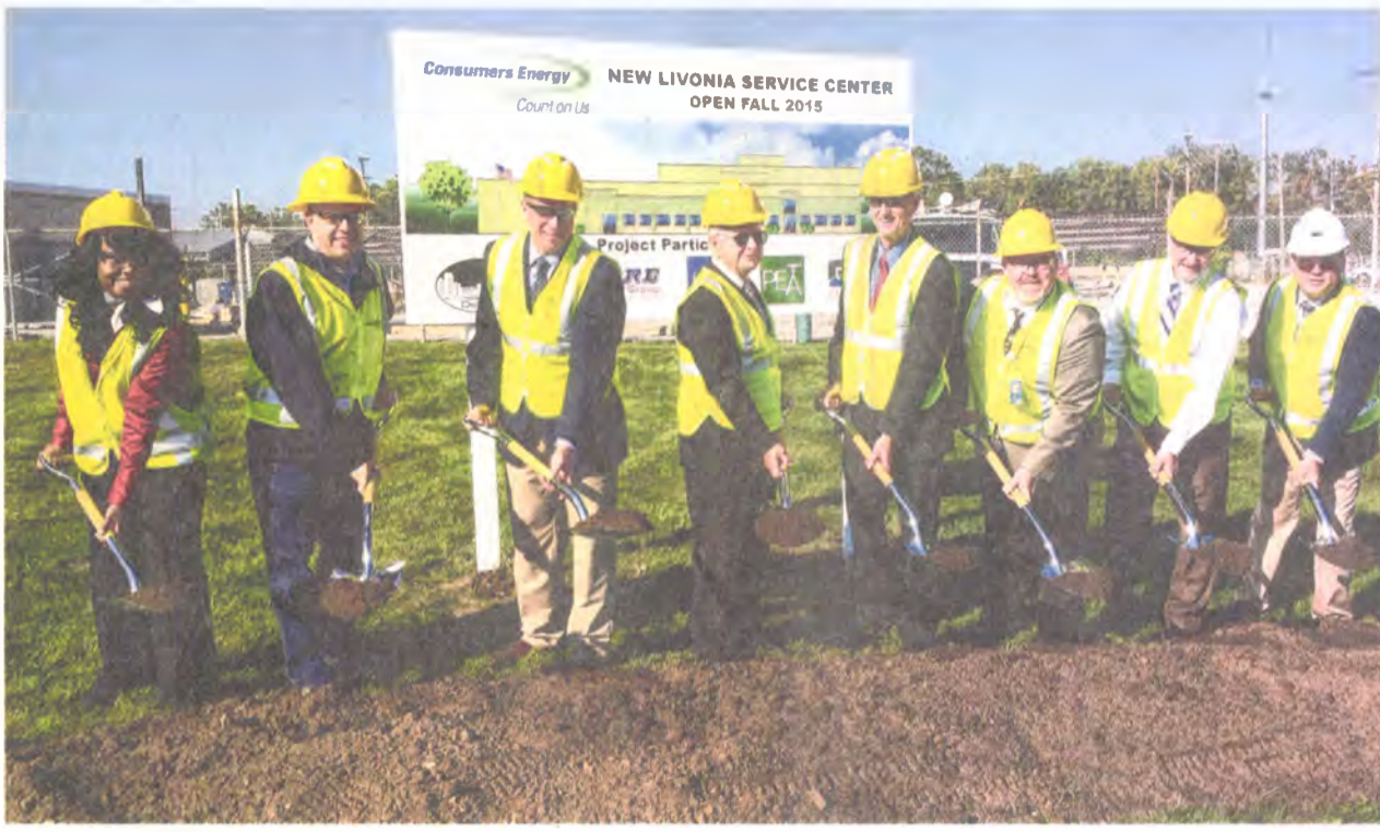
Officials from Consumers Energy, the city of Livonia, Livonia Chamber of Commerce and DeMaria take part in the groundbreaking for the new Livonia service center.
