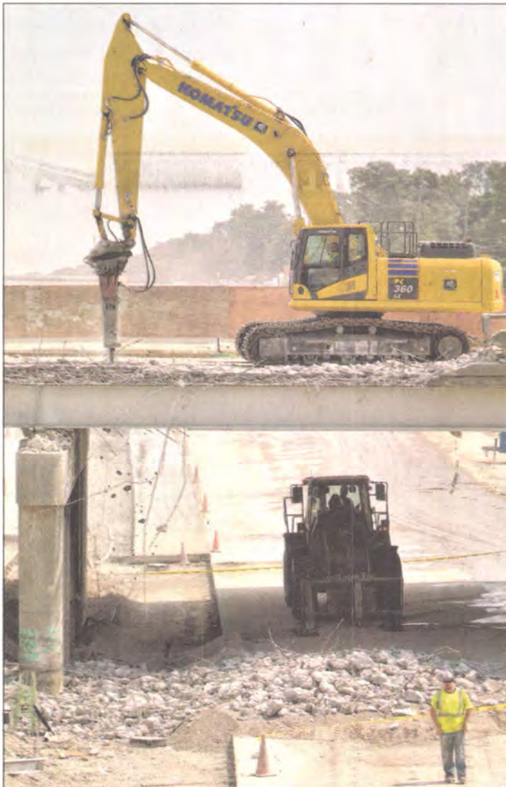
The road surface and side walls of the Beech Daly bridge are demolished, then rebuilt.
