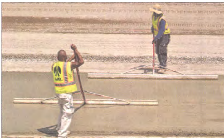
Some hand-finishing is required before the concrete sets.
