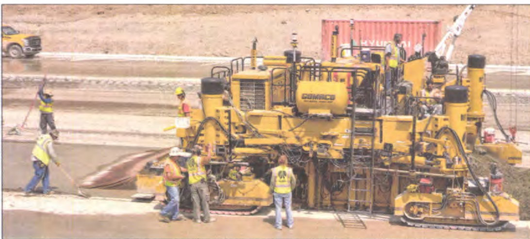
Miles of concrete are laid by machines like this. Mixed concrete is dumped in the path of the machine, which spreads and finishes the mix. PHOTOS BY BILL BRESLER | STAFF PHOTOGRAPHER
