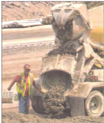
A constant stream of trucks dumps concrete that will become finished road surface, in a matter of minutes.
