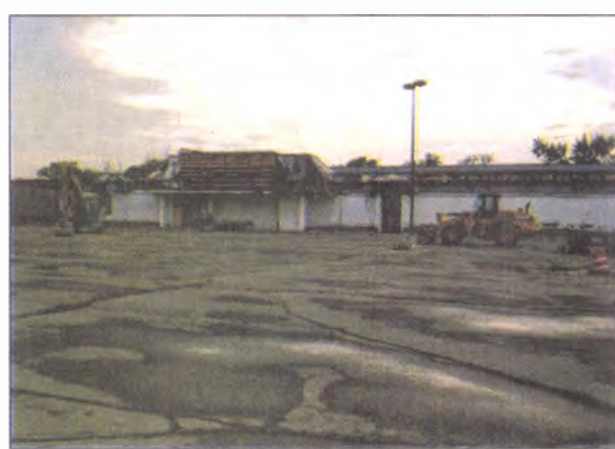
Crews are demolishing the long-closed Service Merchandise store on Nankin Boulevard.
