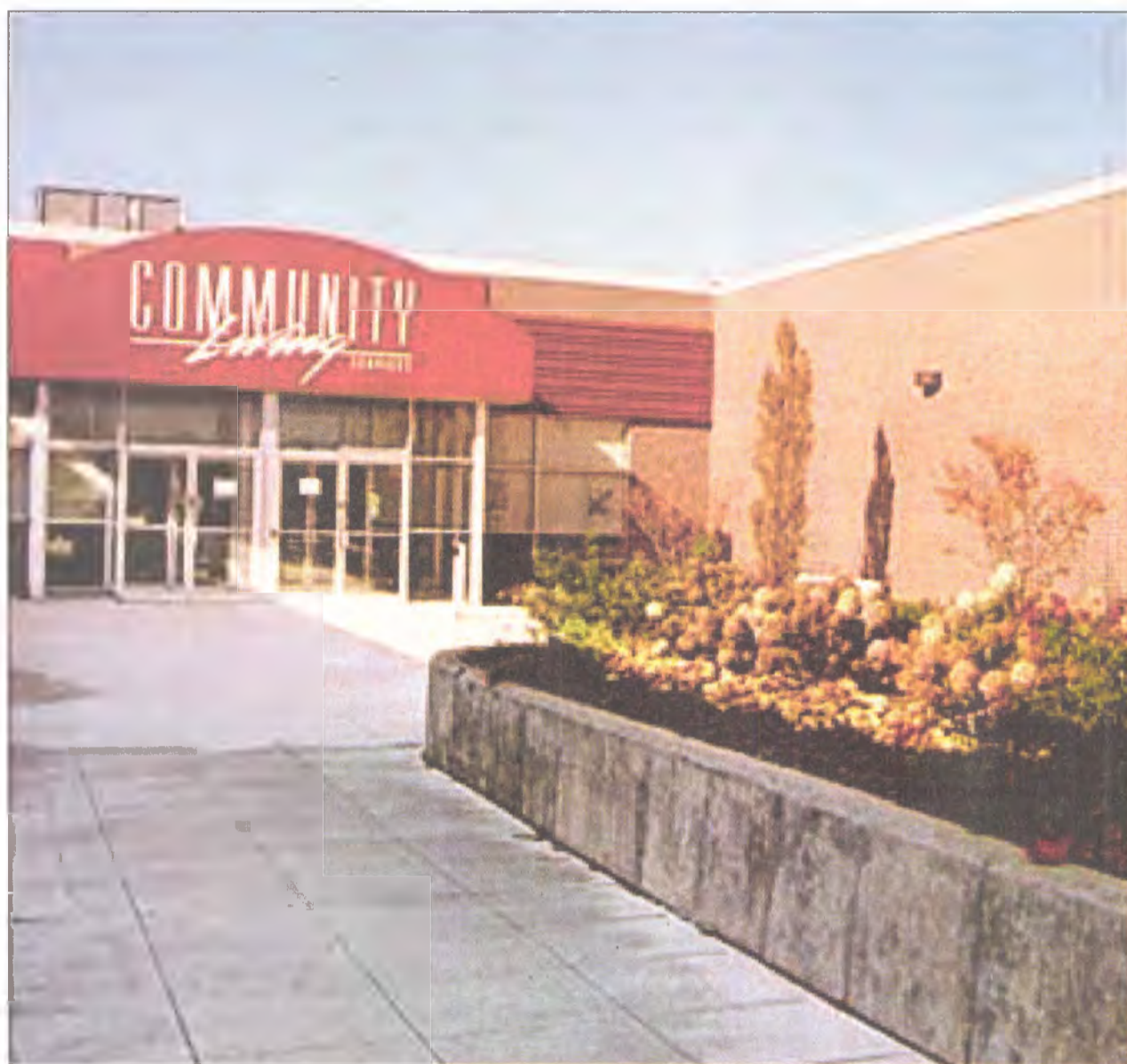
Improvements at CLS in Wayne have included landscaping the courtyard and parking lot island and adding awnings and new doors.
