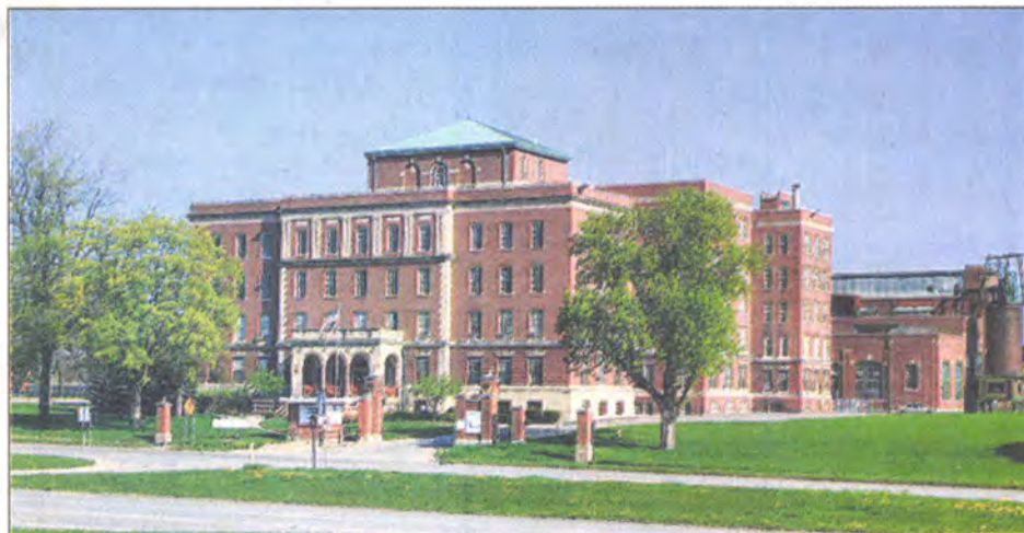
The Kay Beard Building, which has housed the Eloise Museum, is slated to be closed this year by Wayne County. That building, the bakery, fire house and power plant are all that remain of the former infirmary and asylum.
