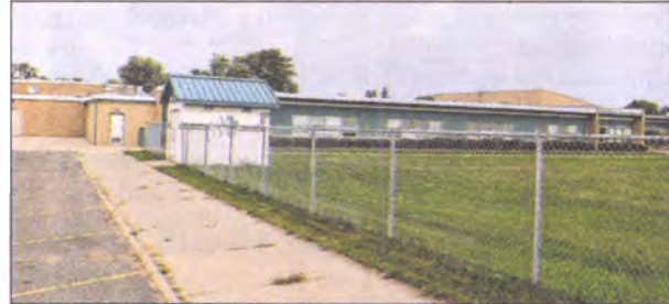
Nankin Mills school is at 8100 Hubbard, at the corner of Ann Arbor Trail, in Westland. It is not part of the historic Nankin Mills properties just to the west.
