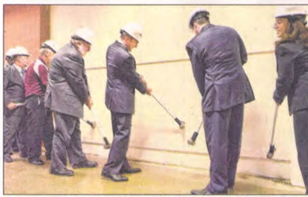
Westland Mayor William Wild (center) and members of the city council take swings with sledge hammers at a wall inside the former Circuit City building to symbolize the groundbreaking for the new Westland City Hall. FILE PHOTO
