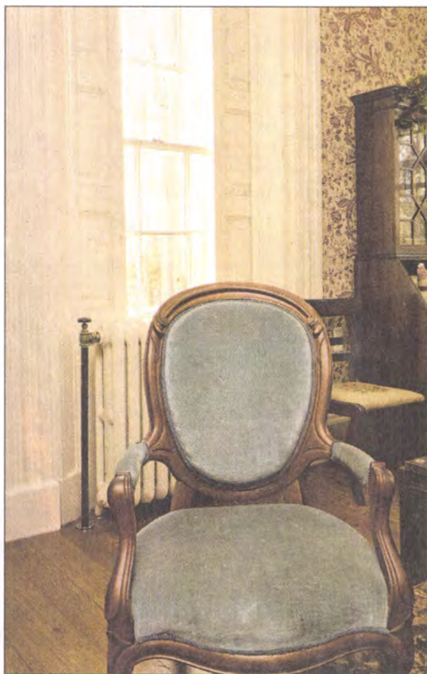
Note the built-in shutters on the window that slide back into the wall. The shutters had been painted in. The carpenters refurbishing the windows discovered and restored the pocket shutters to good working condition.
