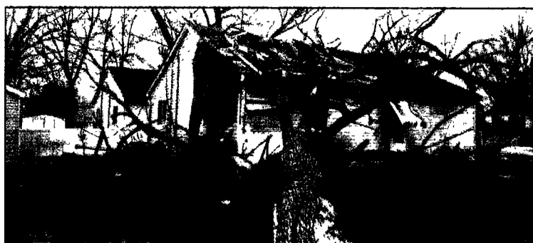
A tree fell on a house in the 29900 block of Balmoral in Garden City during the Sunday's severe weather. GARDEN CITY FIRE DEPARTMENT
